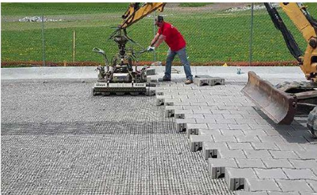
PaveDrain Parking Lot Installation, Cedar Rapids, IA Credit: Besser Company
