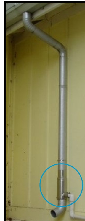
Fig. 9: Downspout filter
