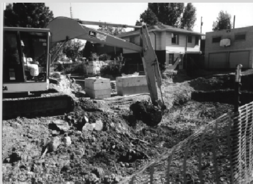
FIGURE 7.2 Excavation of uranium mill tailings from a residential septic system, Grand Junction, Colorado, 1993. SOURCE: U.S. DOE Office of Environmental Management.
