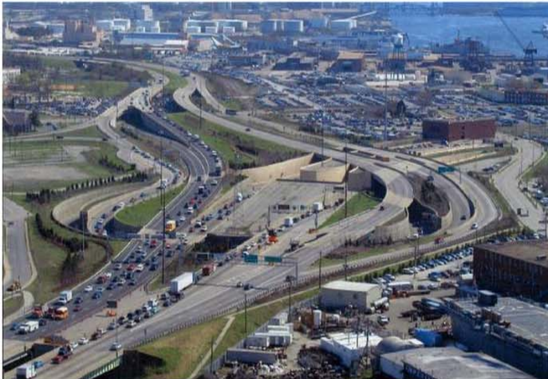
ERT – Downtown Tunnel – I-264
