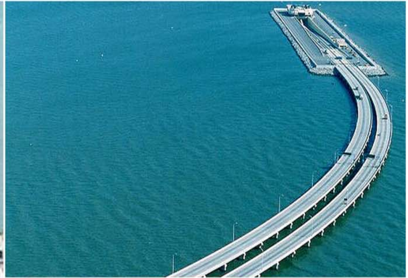
Monitor-Merrimac Memorial Bridge-Tunnel I-664
