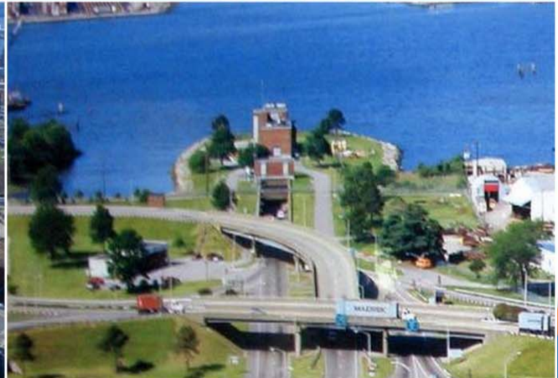
ERT – Midtown Tunnel – U.S. Route 58
