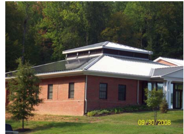
20KW Roof Mount Solar, Marathon Building
