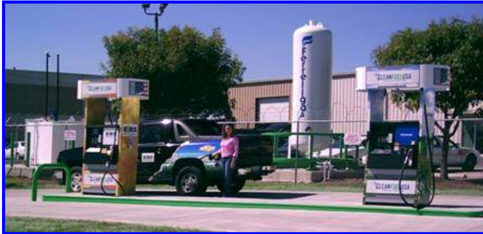
Example of a government fleet fueling facility in San Antonio TX. The fleet pumps are inside the fence. The alternative fuels, pictured, are publicly accessible.
